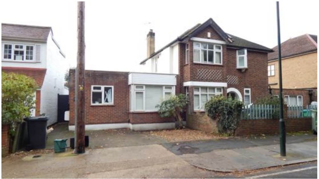
Image 02 - Front elevation - No175A in centre, No173 at left, No175 at right.
