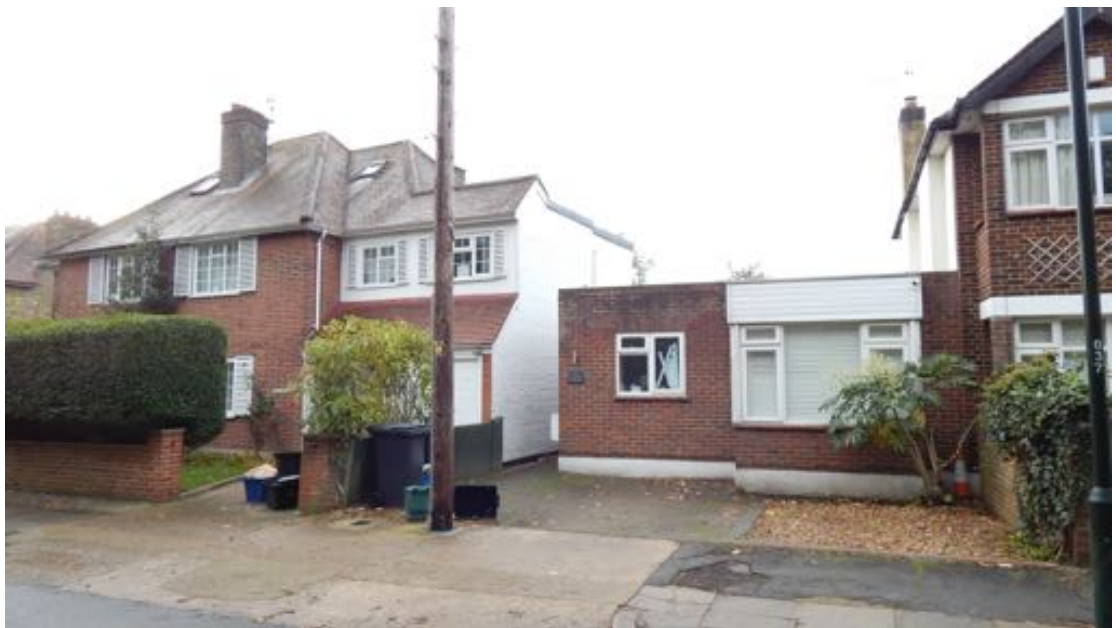
Image 01 – Front elevation – No175A in centre, No173 at left, No175 at right.
