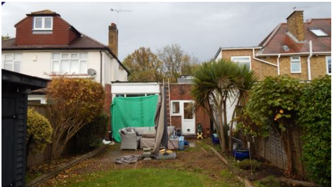
Image 03 - Rear elevation - No175A in centre, No175 at left, No173 at right.
