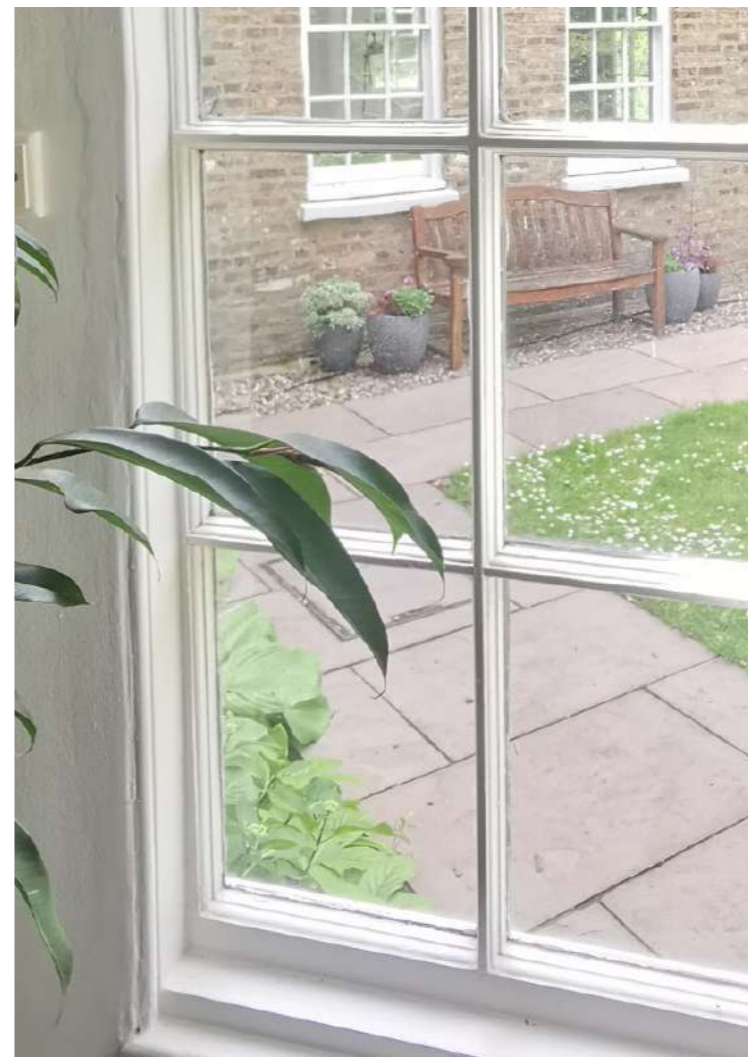
W-022-17 INTERNAL GLAZING BAR DETAIL
