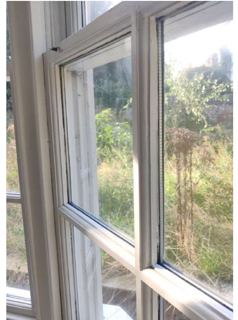
INTERNAL GLAZING BAR DETAIL
