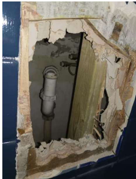
Modern plumbing closed up
