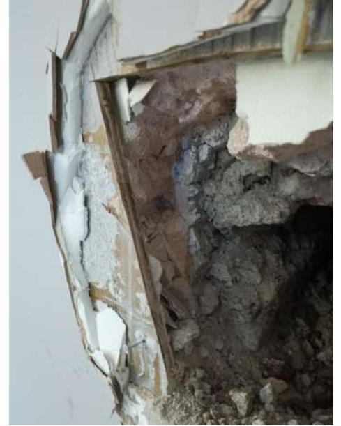
Chimney breast opening
