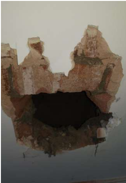
Chimney breast opening
