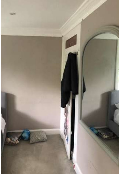
Chimney breast to the right
