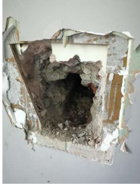
Chimney breast opening
