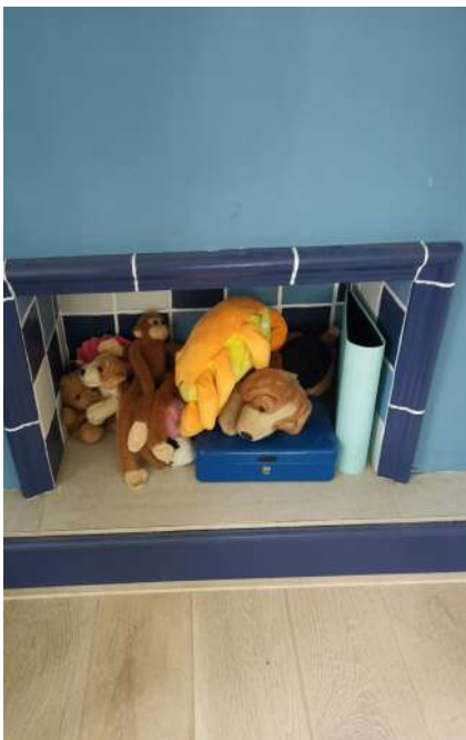
Fire box clad with modern tiles
