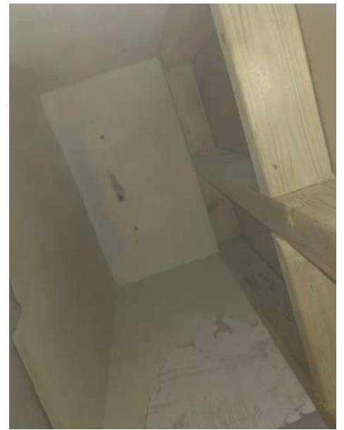
Modern stud structure inside
