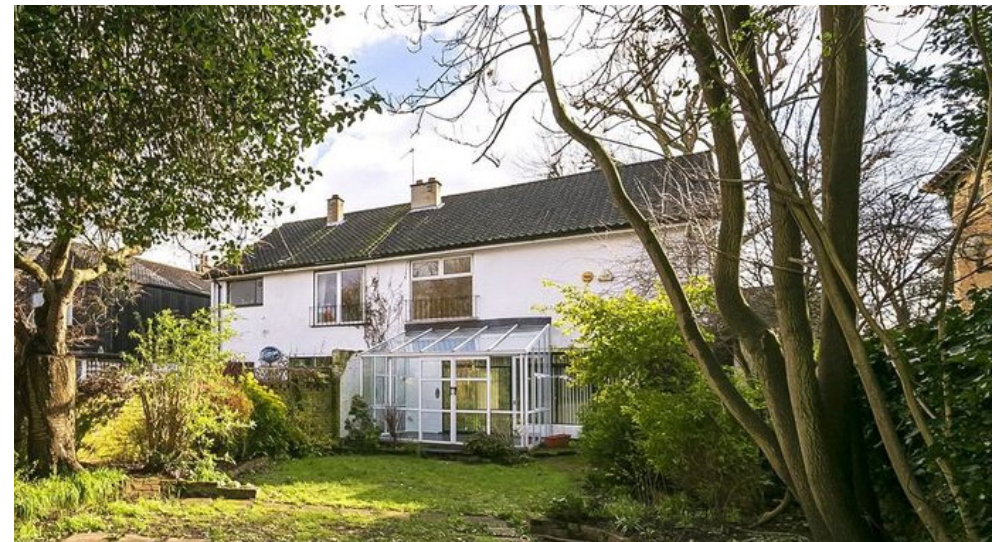
Rear View of the Property
