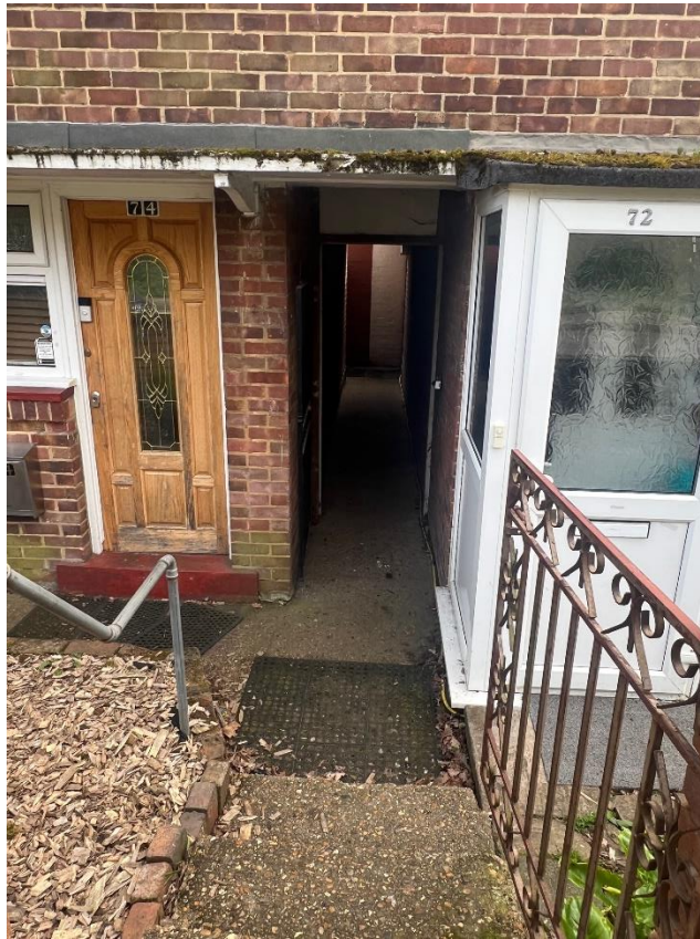
Photograph 3 (08/04/2024) View of the pedestrian access to the rear property.
