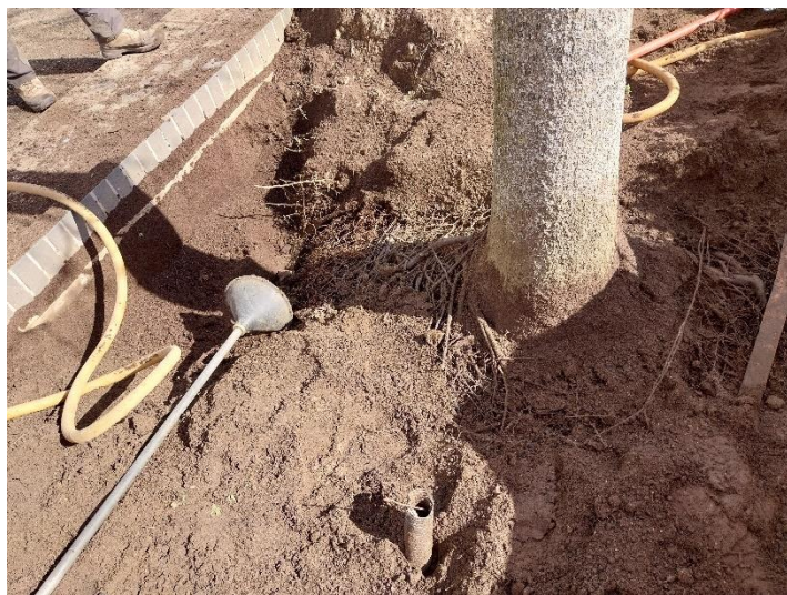
View mainly of north side of rooting area
