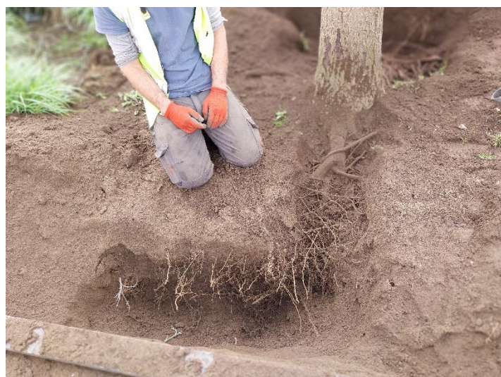
View of the root ball on the north side where it has not grown out towards the hard standing
