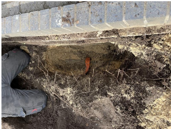
View of the north site of the rooting area showing roots growing towards the wall within the sand but not dense and dry and brittle
