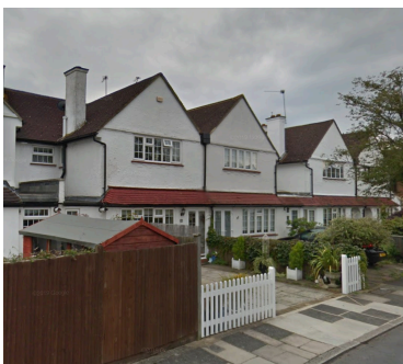
Terrace general view
