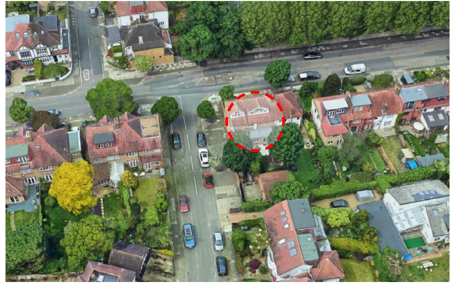
bird's eye view of the site looking west
