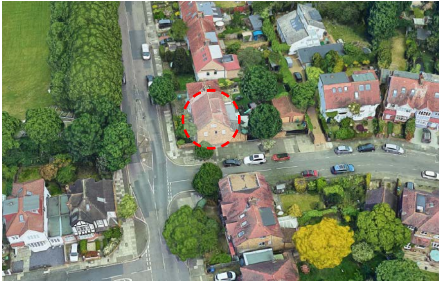
bird's eye view of the site looking north
