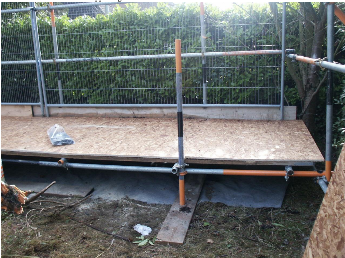
Photo 2 Scaffold framework supporting wooden boards
