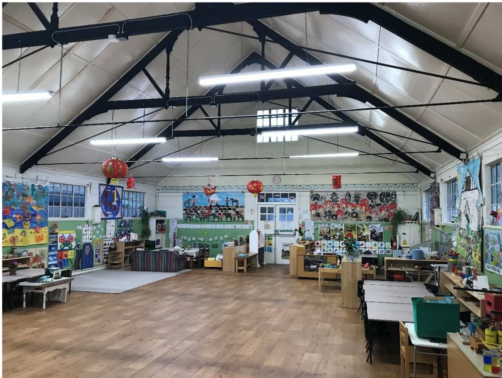
Internal view showing the existing trusses with additional tie rods
