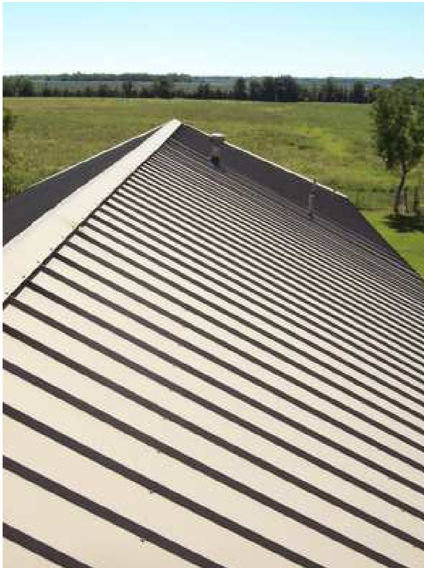
Image of an Aluminium Standing Seam Roof, in a lead grey colour
