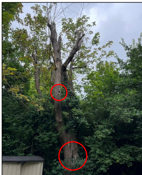
T5/945 Norway maple - extensive decay in lower stem and main stem sections - circled red
