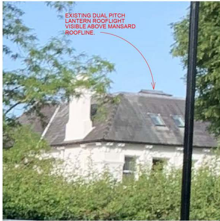
04. Close up extract from View B of 16 St Peters Road roofline.
