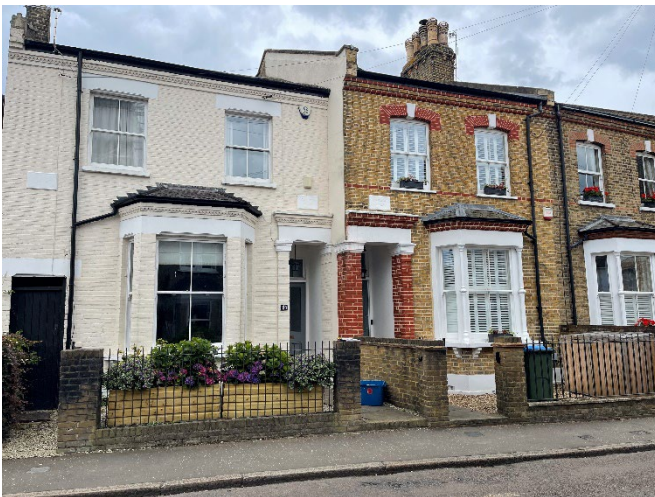
Image showing the front of the property. The fire appliance would need to stop on Oldfield Road outside of the property.
