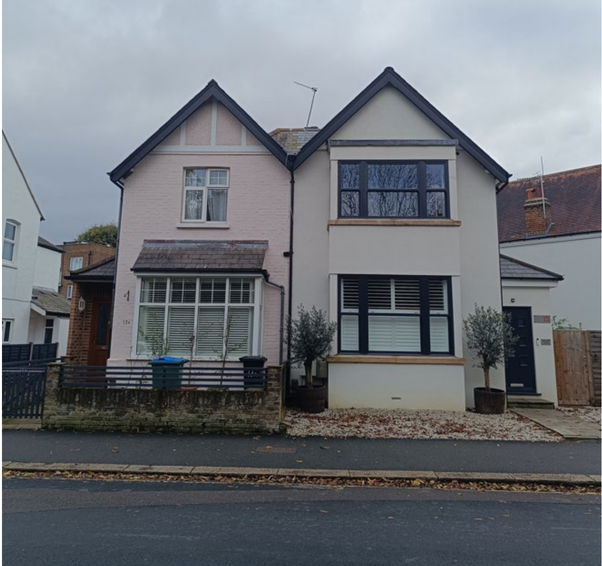
Image 2: Application building (right) (Source: Site visit 29 October 2024)
