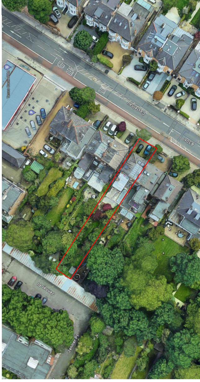
Existing Site View
