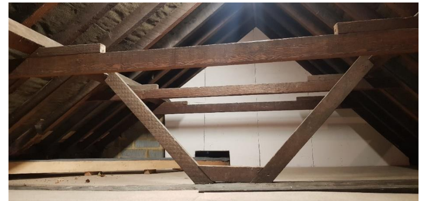
Image 21: Existing Roof Structure
