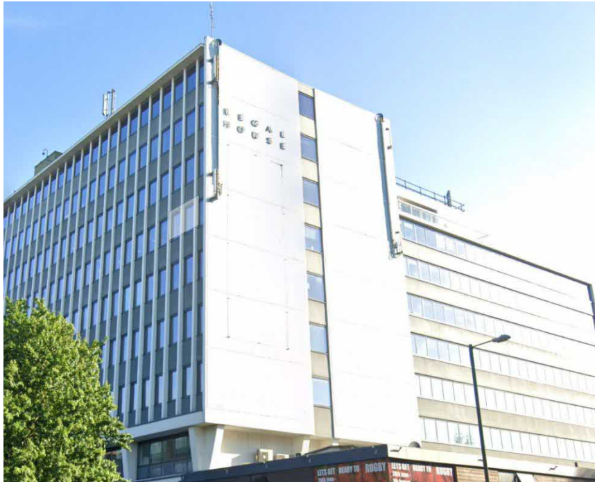
The Southern Flank Elevation of Regal House
