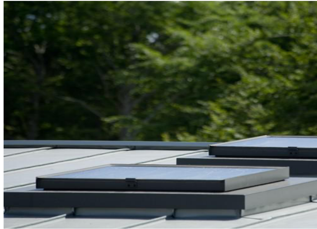
above images: Examples of The Plateau Conservation Rooflight by The Rooflight Company proposed for the existing house new rooflights ( Rooflight Ref: nRL03,04,05 & 06 ) and installed to manufactures recommendations on the proposed new Terne Coated Stainless Steel hipped roof cover.
