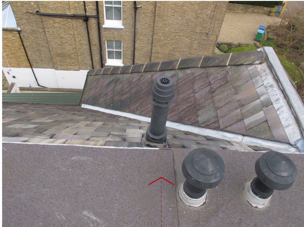
03. Existing Service Vent Pipes (February 2023)
