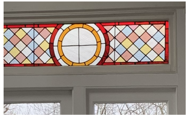
PHOTO OF CONSERVATORY WINDOWS
