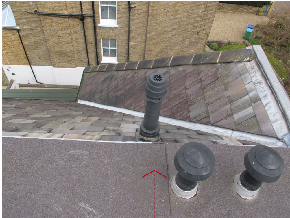
03. Existing Service Vent Pipes (February 2023)
