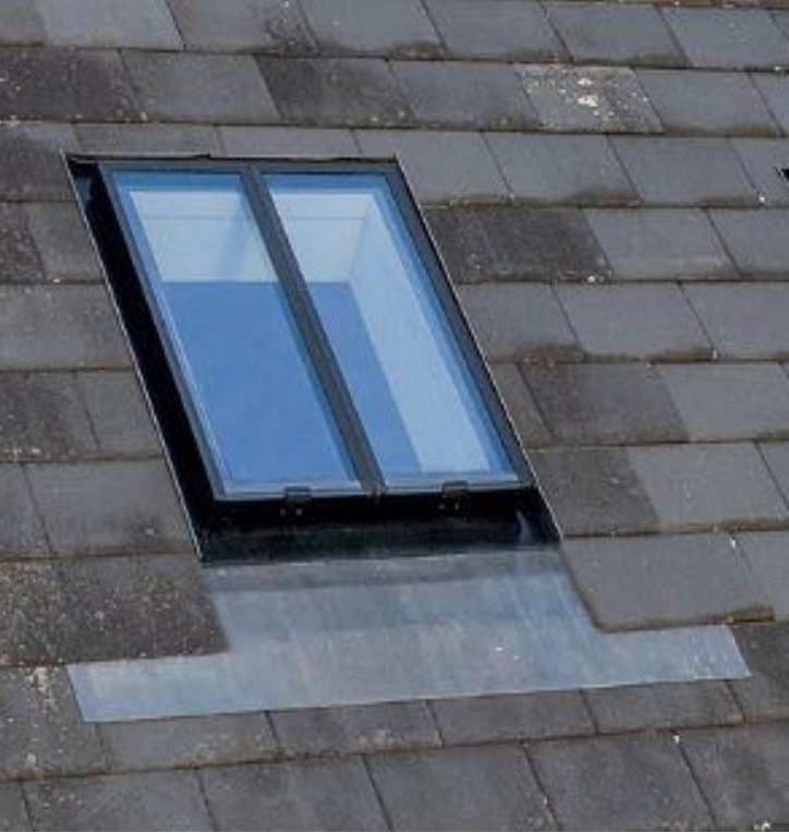
above image: The Original Conservation Rooflight by The Rooflight Company with lead flashing proposed on South West (Front) Elevation slate roof plane.
