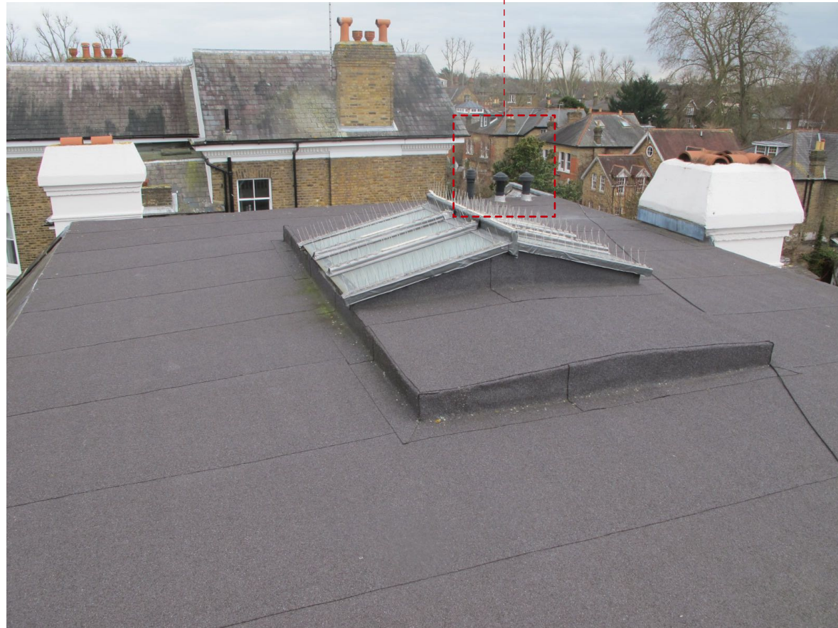
01. Existing Roof looking towards 14a St Peters Road (February 2023)
