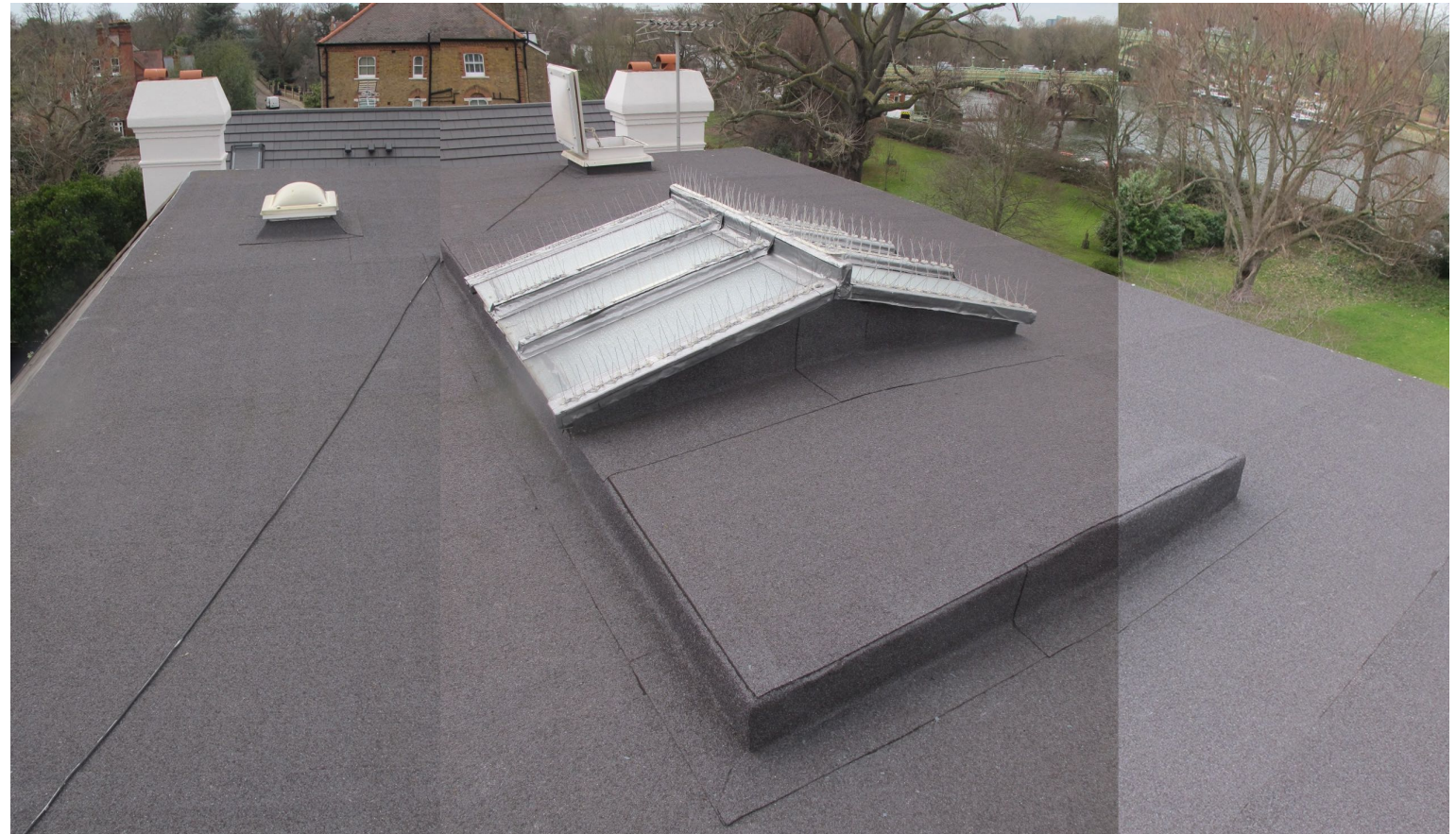
02. Existing Roof looking towards 18 St Peters Road (February 2023)
