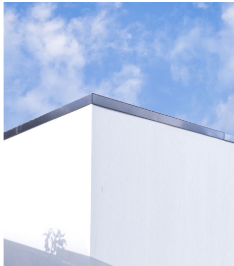
Above image: Example from a single storey modern extension with the same materiality of white painted lime rendered and Terne Coated Stainless Steel parapet coping.
