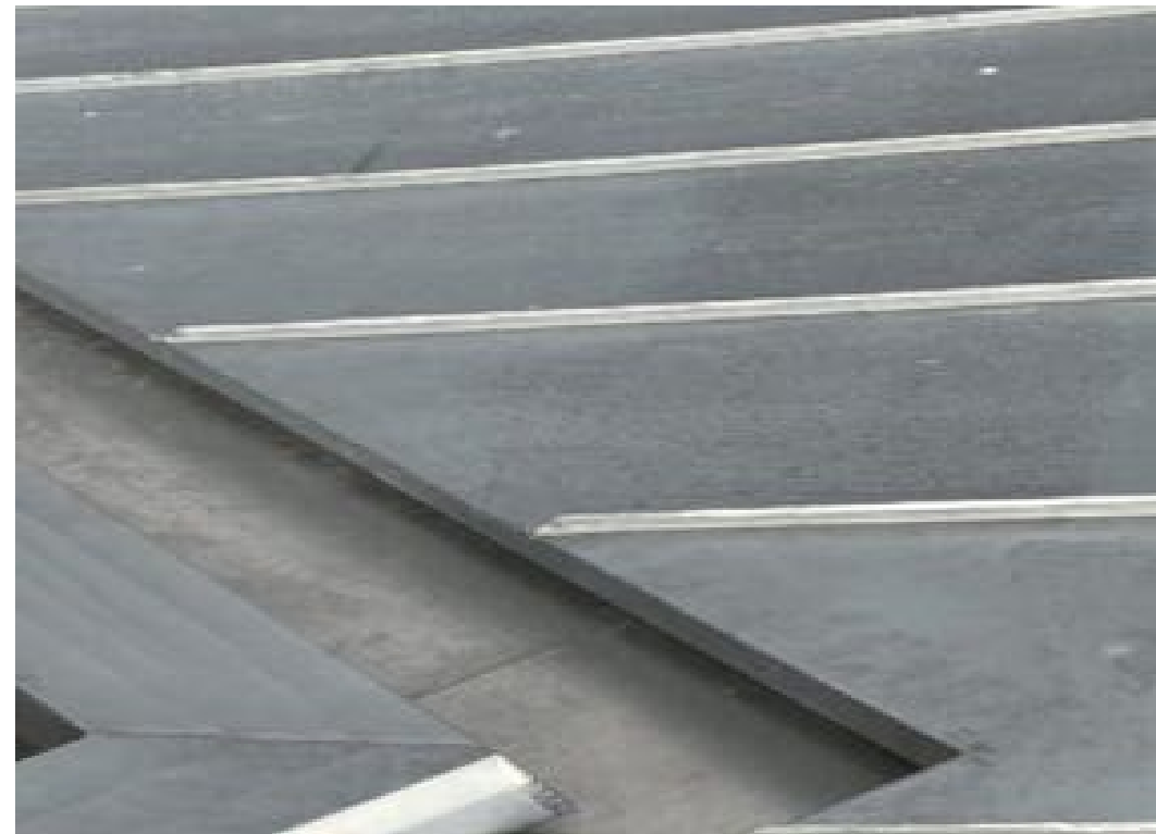
Above image: Example of Terne Coated Stainless Steel concealed gutter parapet, (with folded seams), over white painted render wall as proposed on the new build side extension roof.
