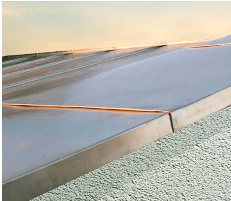
Above image: Example of Terne Coated Stainless Steel parapet, (with folded seams), as proposed to cap the 16 St Peters Road new build side extension's white painted lime render walls.
