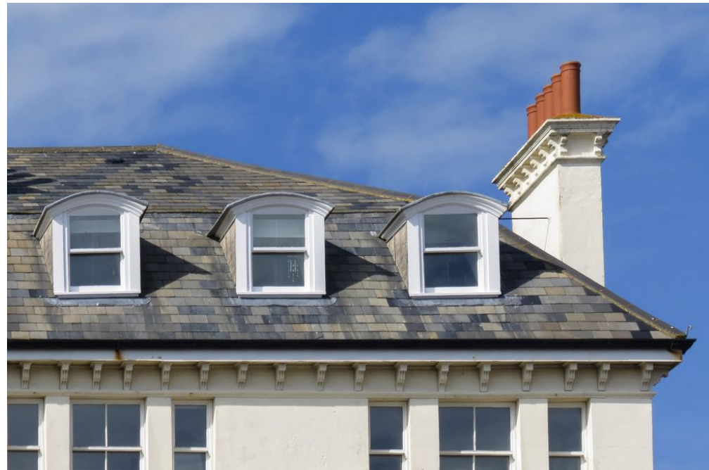
above image: Example of late 19c Victorian dwelling's mansard roof with three dormer windows lead lined cheeks. As per our 16 St Peters proposals the white painted timber box sash windows in this example comprise one over one fenestration. Additionally, their adjacent white timber lining boards provide a stop to the dormer cheek leadwork on the front face to meet the sash window as per our proposed details on BHA drawing Sk42, Sk43 & Sk48 .
