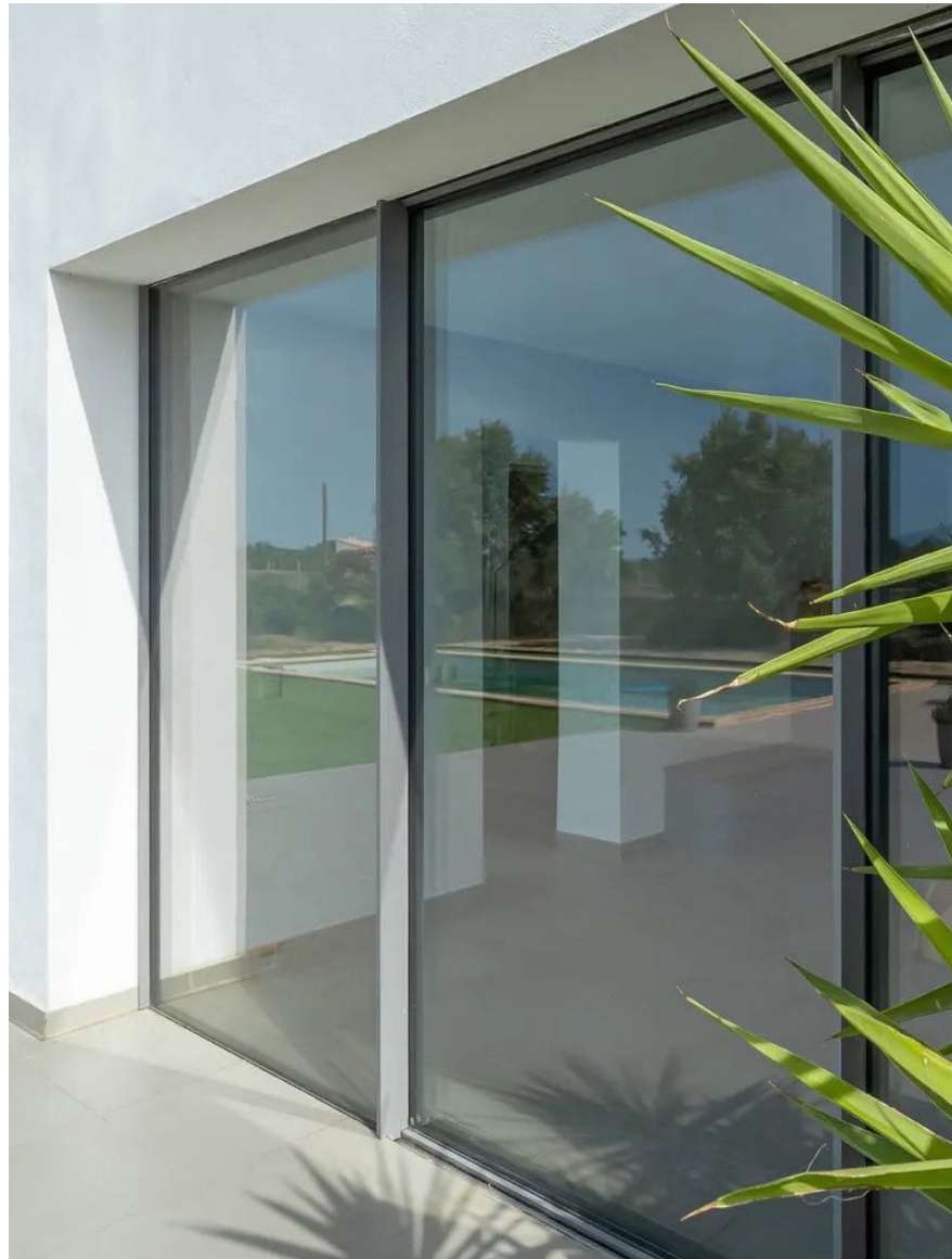
Above image: Close up detail of Sky-Frame Classic brushed stainless steel frameless glazed sliding door system set within a newbuild white lime rendered modern building as proposed on the rear garden elevation of the new extension.
