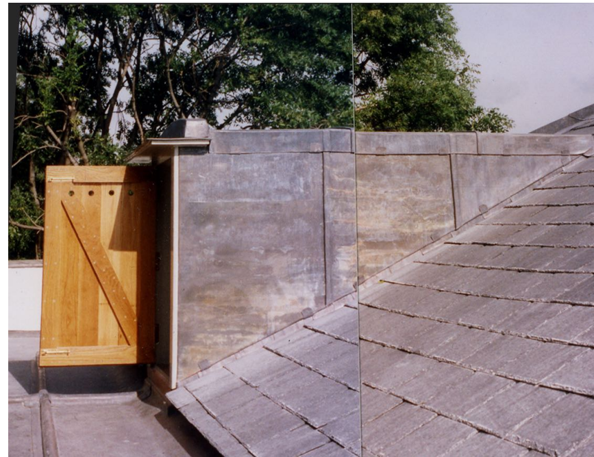
above images: Example from a previous Butler Hegarty Architects project of the proposed leadwork roof and cheeks to be used on the three new 16 St Peters Road dormer windows including the lead lined curved hood eaves above the sash window. This example also shows the proposed corner junction detail between the dormer cheek leadwork and white painted timber lining boards.
