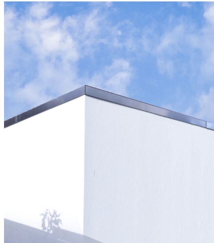
Above image: Example from a single storey modern extension with the same materiality of white painted lime rendered and Terne Coated Stainless Steel parapet coping.
