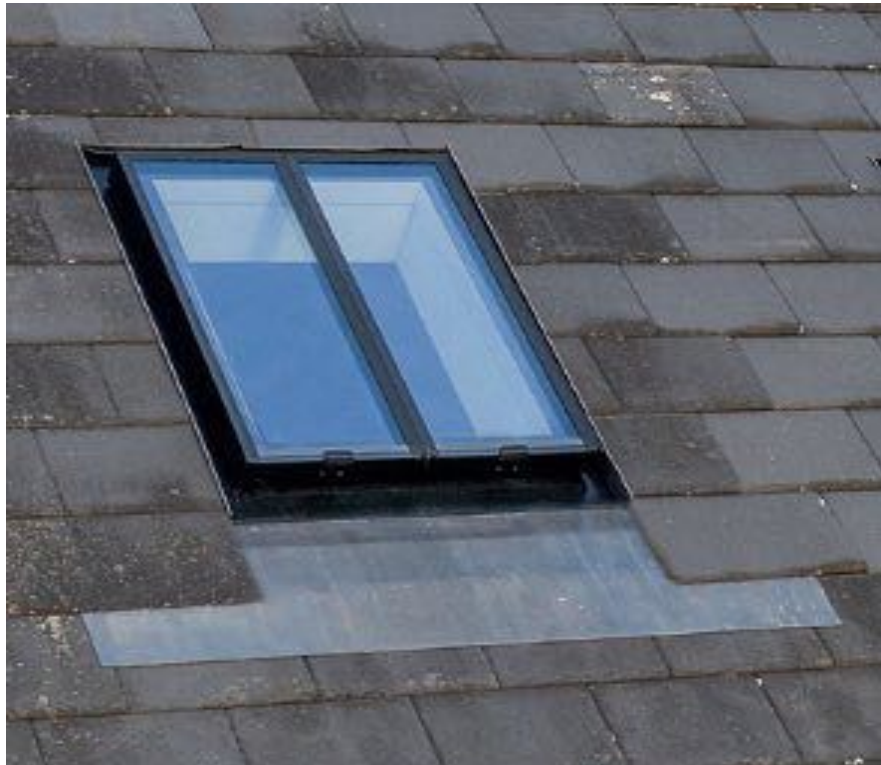
above images: Examples of The Original Conservation Rooflight by The Rooflight Company with lead flashing proposed on South West (Front) Elevation ( Rooflight Ref: nRL02 ) for the second floor Bathroom 2R7 and installed to manufactures recommendations to finish flush with the existing pitched slate roof.
