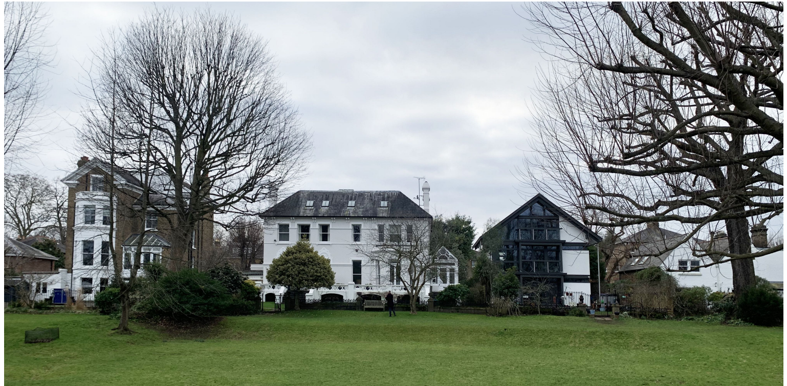
04. Existing Rear Elevation from Younique Gardens (February 2023)
