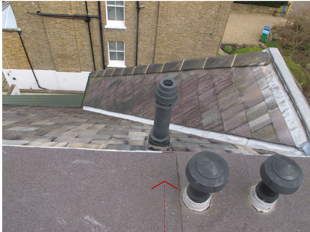
03. Existing Service Vent Pipes (February 2023)
