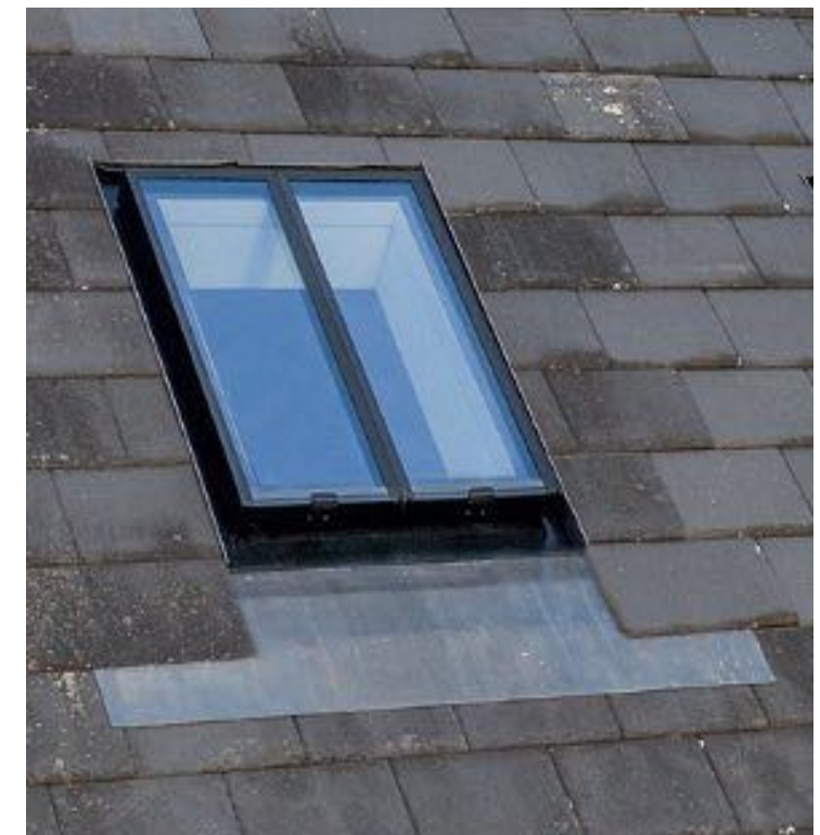
above image: The Original Conservation Rooflight by The Rooflight Company with lead flashing proposed on South West (Front) Elevation slate roof plane.
