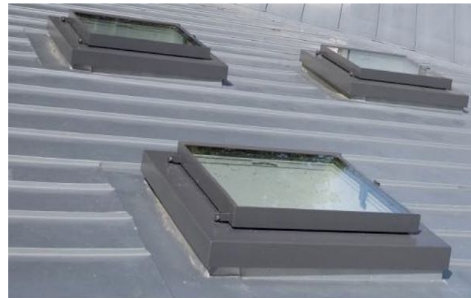
above image: The Plateau Conservation Rooflight by The Rooflight Company proposed for the existing house new rooflights (Rooflight Ref: nRL03,04,05 & 06)
