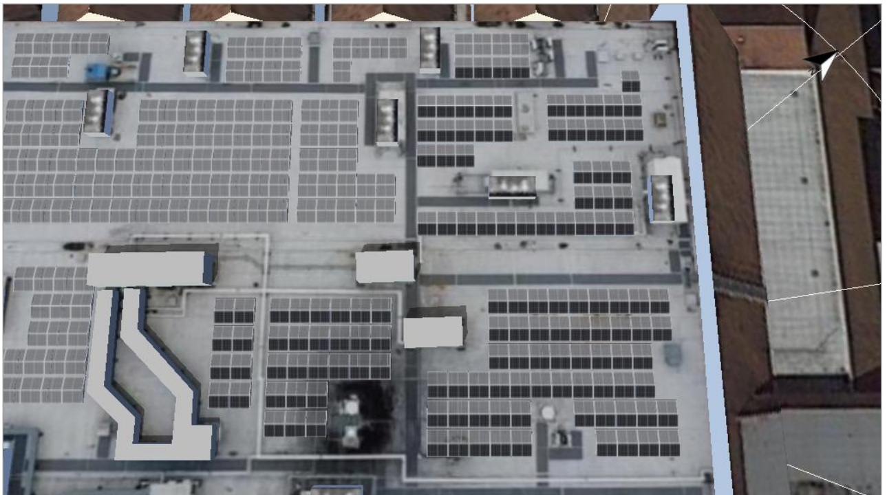
Figure: 3. Module Area - Building 01-Module Area Southeast
