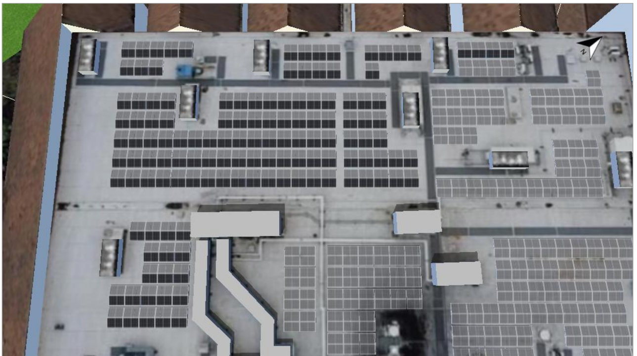
Figure: 1. Module Area - Building 01-Module Area Southeast
