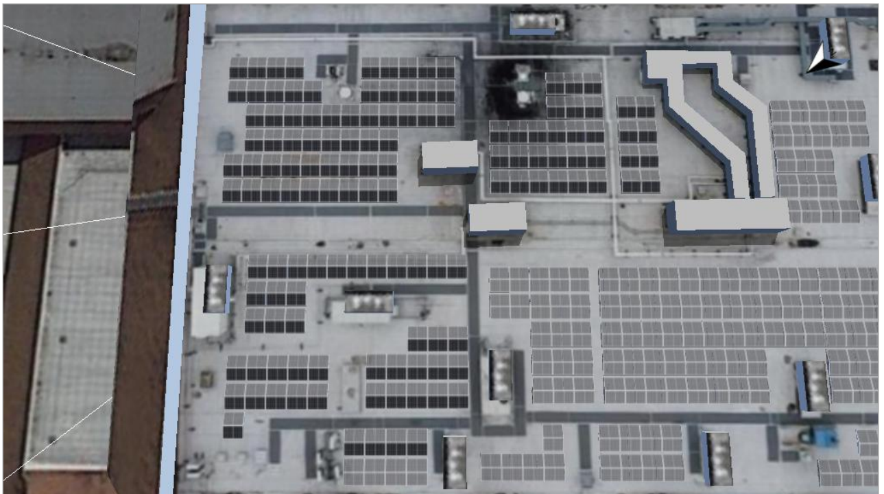
Figure: 4. Module Area - Building 01-Module Area Northwest
