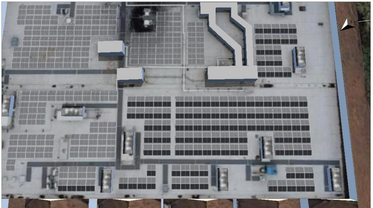
Figure: 2. Module Area - Building 01-Module Area Northwest
