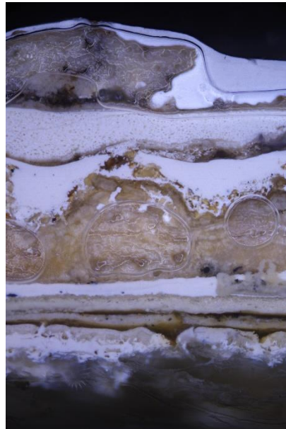
Sample 13 – South elevation, inner side of southern façade, central strut, under side, arris: following test for solubility (positive). Earliest scheme and buff schemes have reacted positively, along with the white paint films showing signs of softening and movement.
