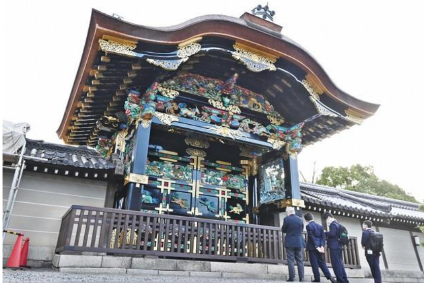
Figure 2: Ornately painted Karamon Gate following a three year restoration, in 2021. (The Mainichi, 2021)
