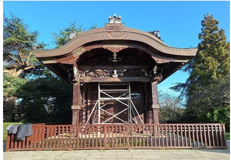
Figure 1: Image taken in January 2024 of the south elevation of the Japanese Gateway.
