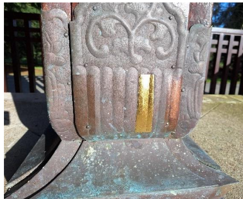
Figure 14: South side of north-eastern post, showing the copper ornamentation test areas.
