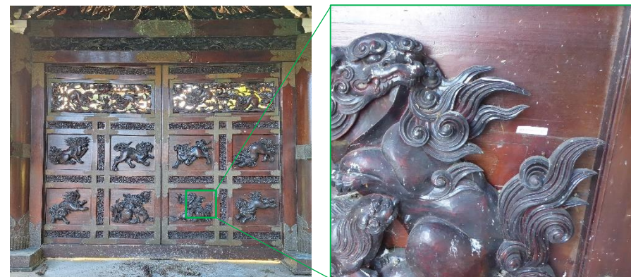
Figure 12: Close up of carved beast on north side of door, showing possible scarring of altered position.
