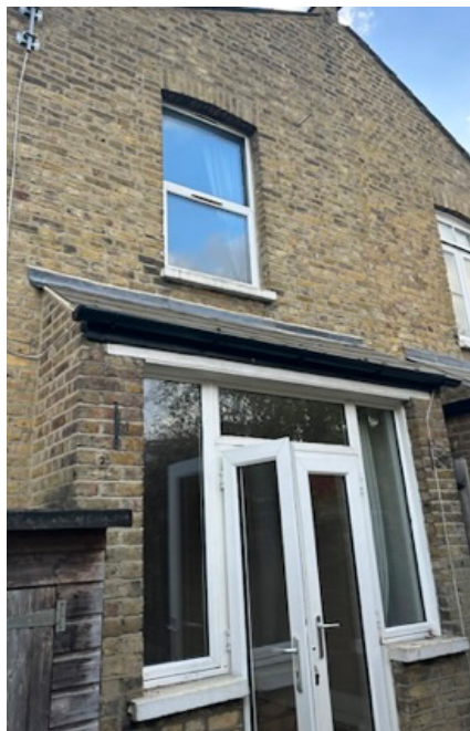
Existing rear view of rear lean-to
