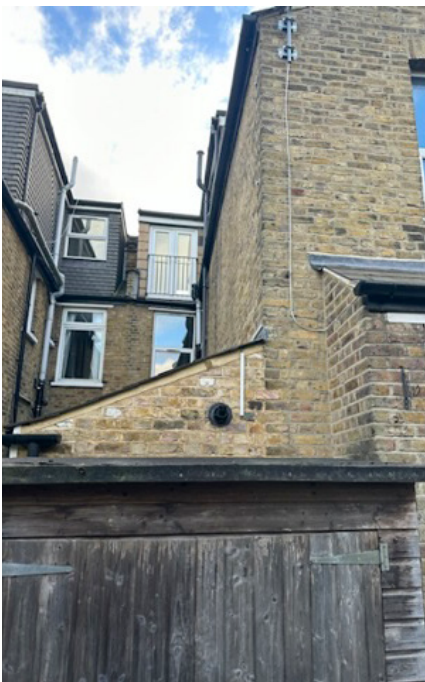
Existing rear view of existing side extension
