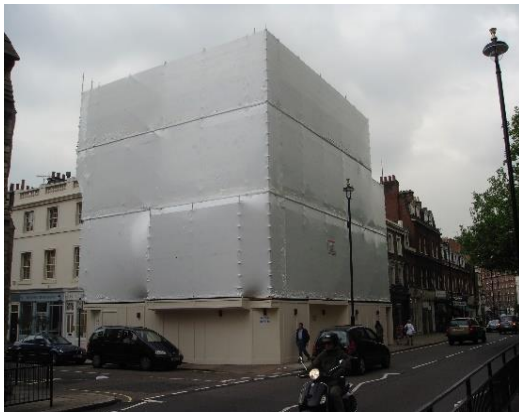
Example of screen protected scaffolding
