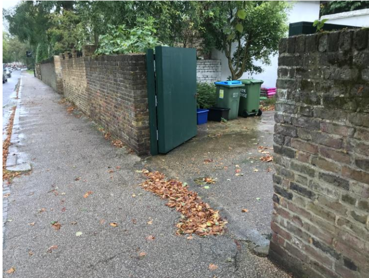
Fig. 03 Existing opening with timber gates
