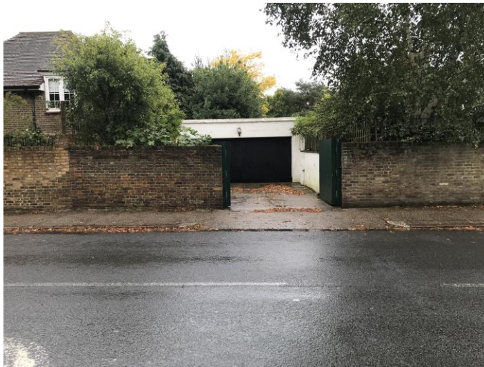
Fig. 02 Existing opening with garage beyond
