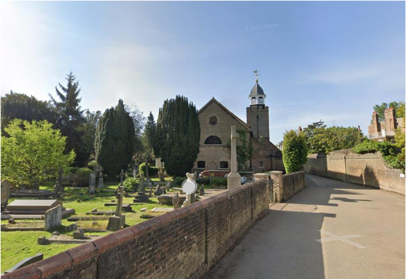
Figure 7 – General view of the Church of St Peter from the north.
