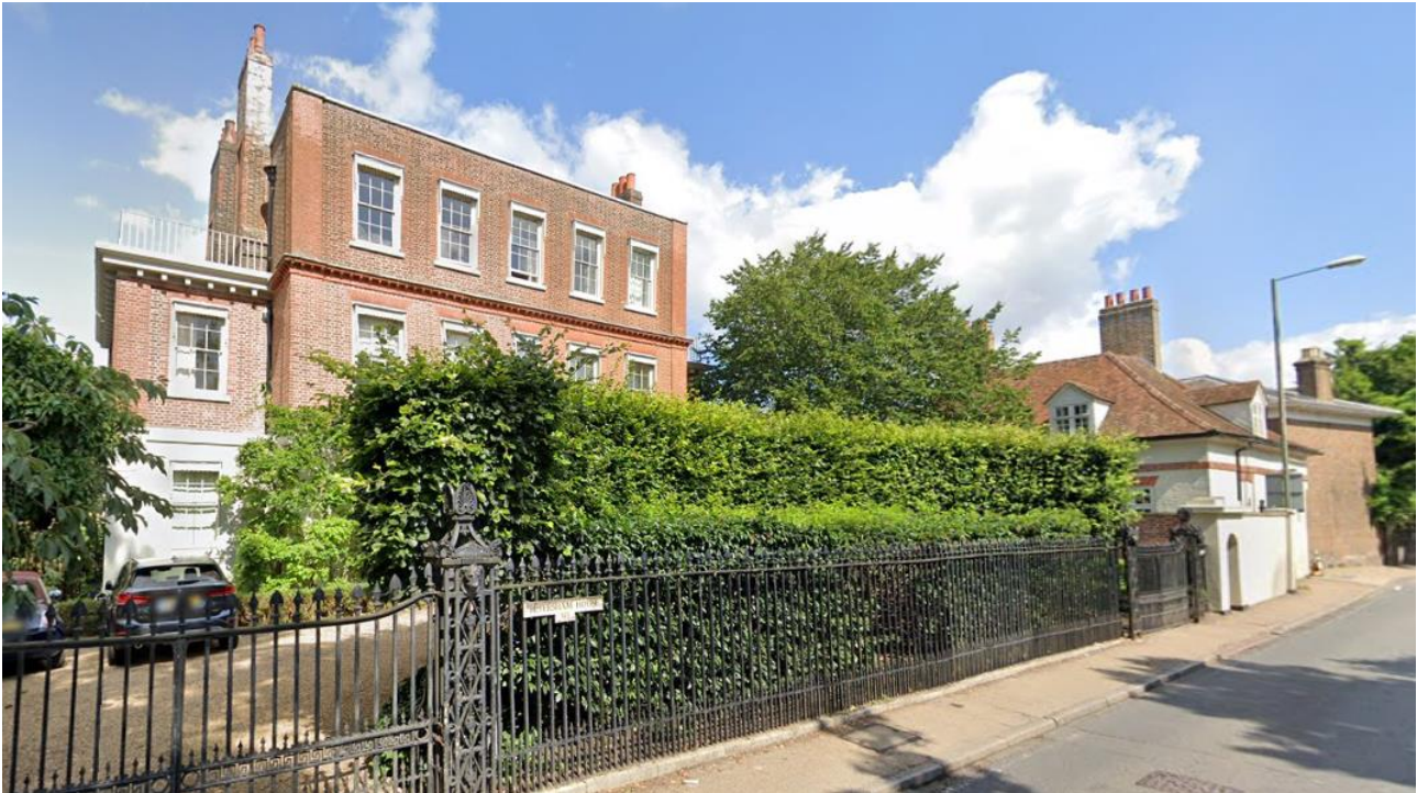
Figure 8 – Petersham House (left), 141 Petersham Road (centre right) and Church House (extreme right) seen looking eastward along Petersham Road.
