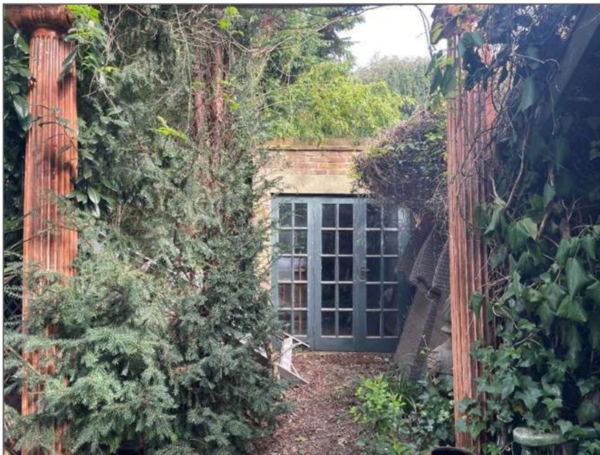
Photograph 5: North-facing view of the garage in the north-eastern corner of the Site, it will be demolished as part of the proposed development.
