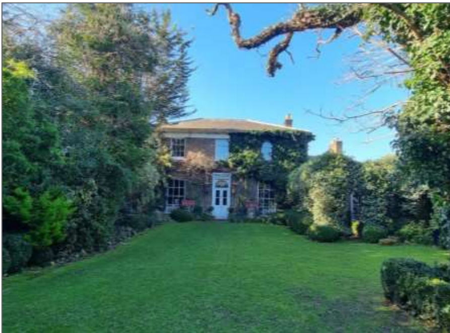
Photograph 3: West-facing view of the main house of 139 Petersham Road, it occupies the western end of the Site.
