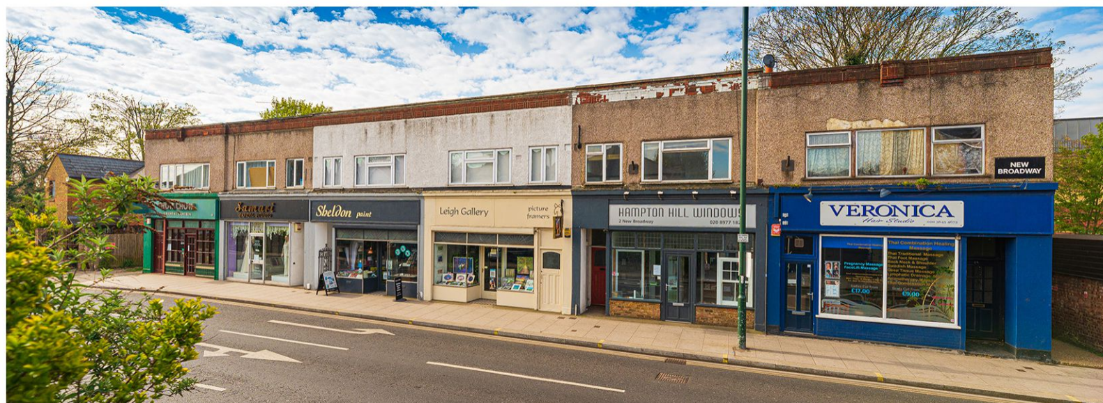
FIGURE 04 - Existing 1-6 New Broadway (no.3&4 in middle)
