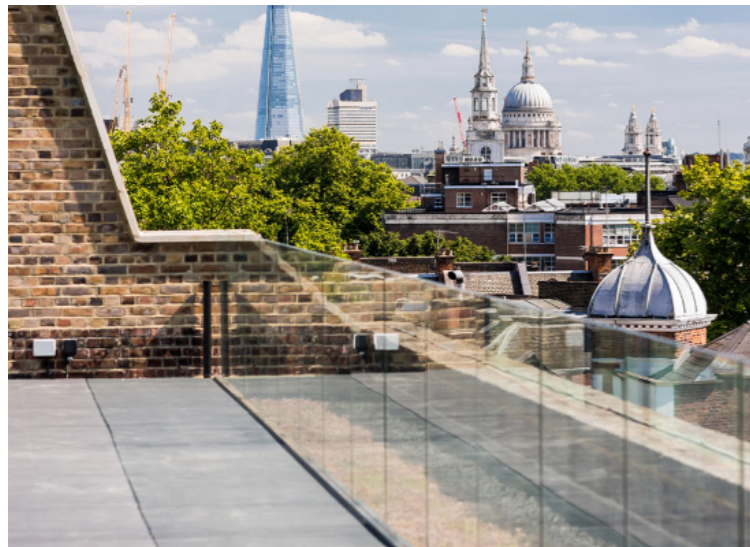
Figure 15 - Frameless glass balustrade example
