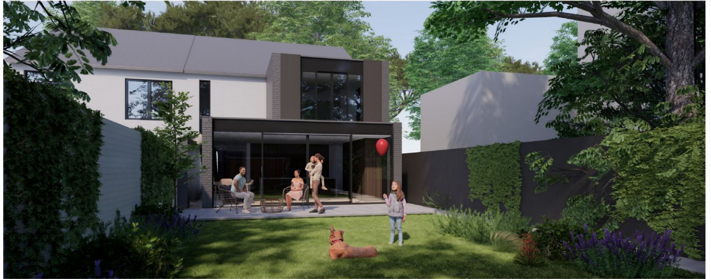
Ground Floor Extension
