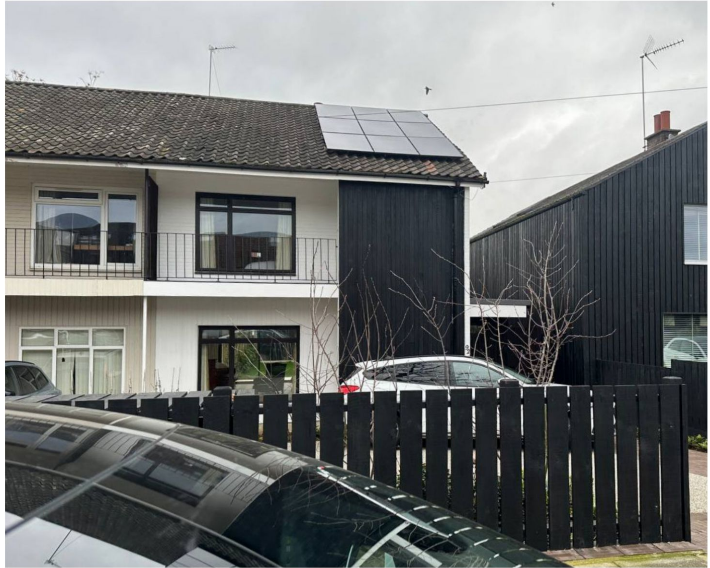
Front View of the Adjacent Property
