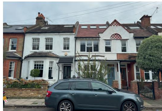
Figure 23: 11 and 13 Ellison Road (east side)
