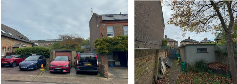
Figure 4: Existing garage fronting onto Ellison Road and the rear of the garage
