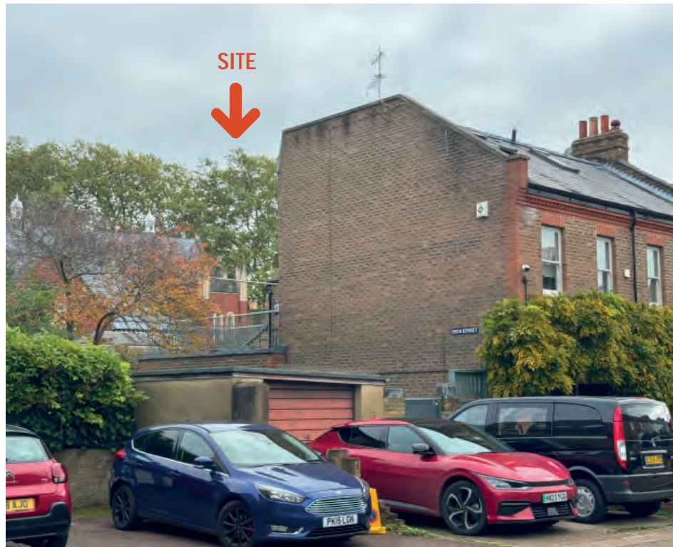
4 Photo view of site with flank wall of 5 Ellison Road beyond.
