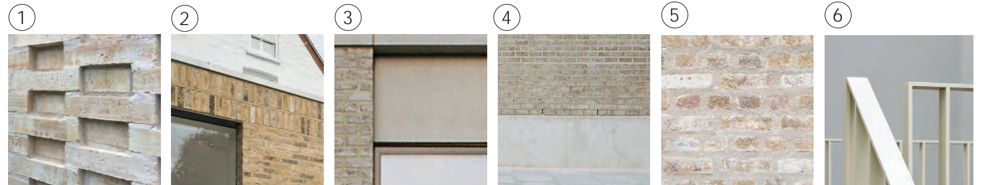
Recessed Brick Detail
