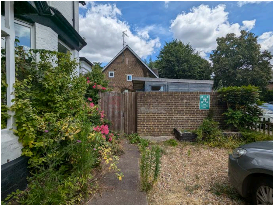
Existing Summerhouse on Front Boundary
