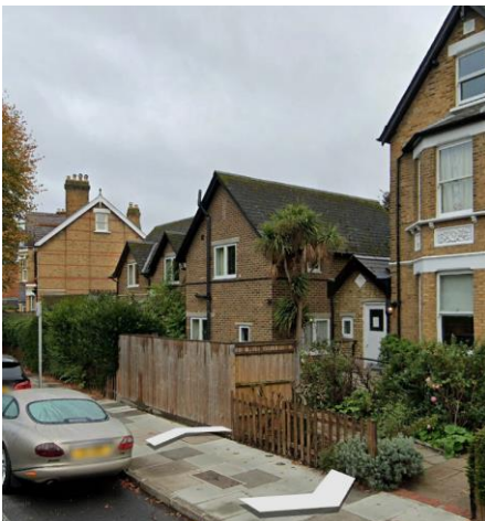
Above – Modern two storey linked building at the western end of the site
