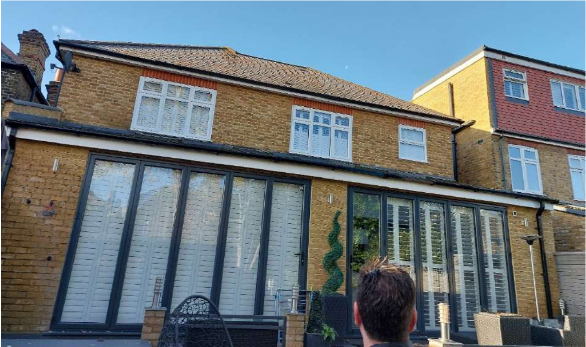
Rear of 35 Elmsleigh Road
