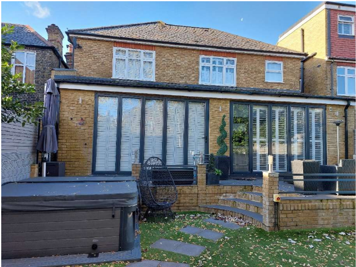
Rear of 35 Elmsleigh Road
