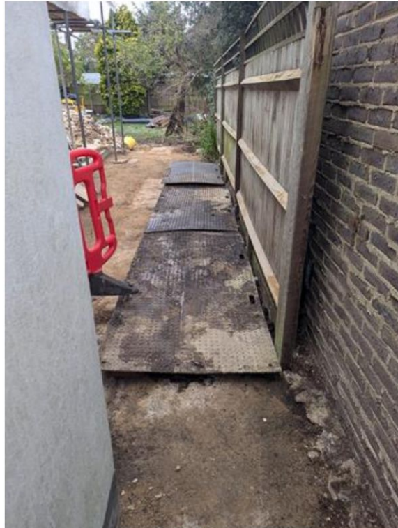
Photo 4. Temporary ground protection over the RPA of T1 [photo CS 22.11.24]
