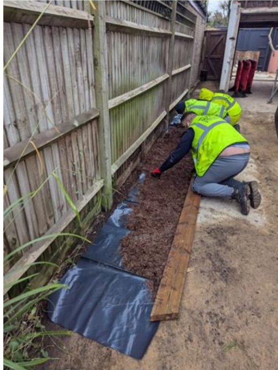
Photo 4. Temporary ground protection over the RPA of T1 [photo CS 22.11.24]
