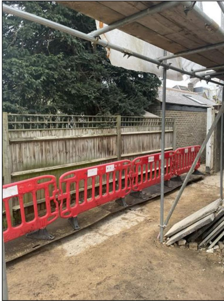
Photo 5. Tree protection fence adjacent to the RPA of T1 [photo CS 22.11.24]
