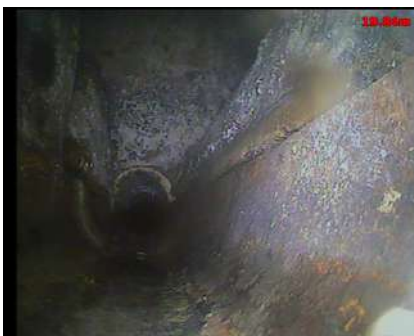
Observation [9]: ENTERS MANHOLE POSSIBLY no30 or 28
