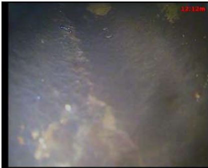
Observation [7]: End Point: RAIN WATER GULLY
