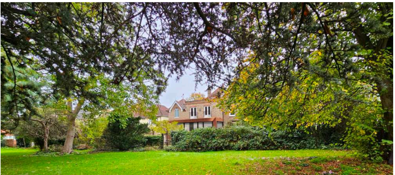
Fig 22: Proposed view of the rear of the house from the trust ground.
