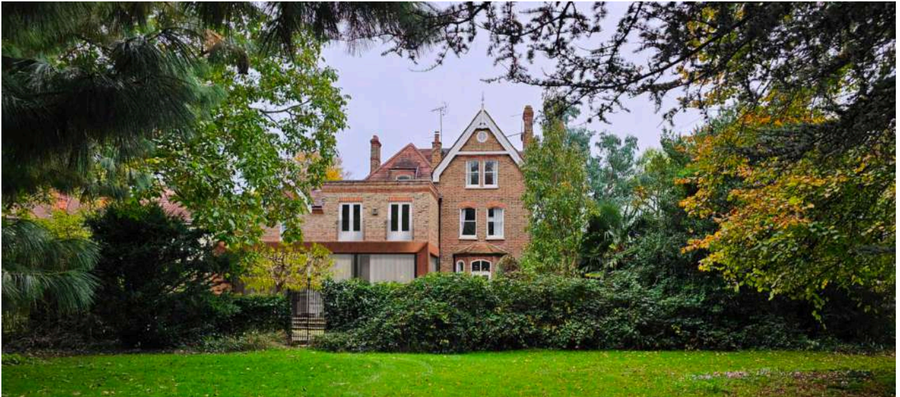
Fig 20: Proposed view of the rear of the house from the trust ground.
