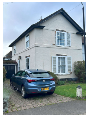
No. 10 Grove Terrace
