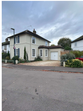
No. 26 Grove Terrace
