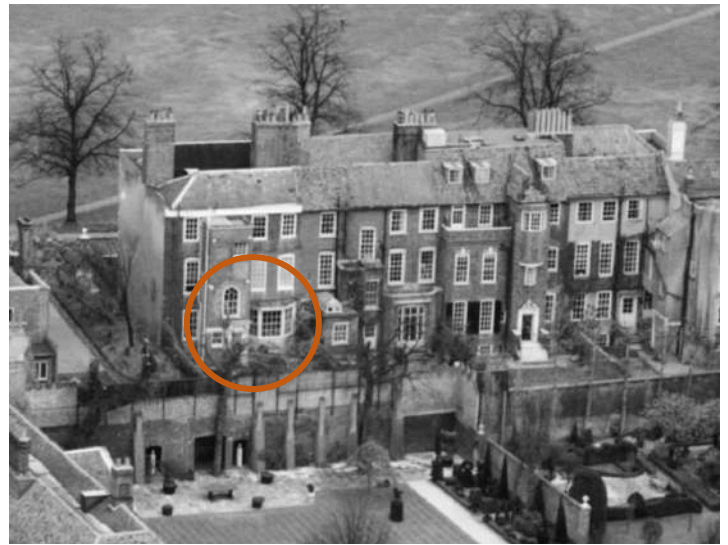
1948 – Ground floor of outrigger infilled. Arched window at first floor level of outrigger.
