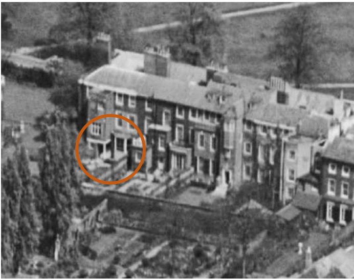
1930 – Open area at ground floor of outrigger. Rectangular window at first floor level of outrigger.
