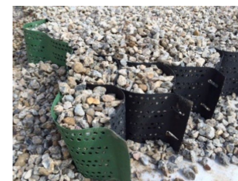
Cellweb, cellular confinement system
