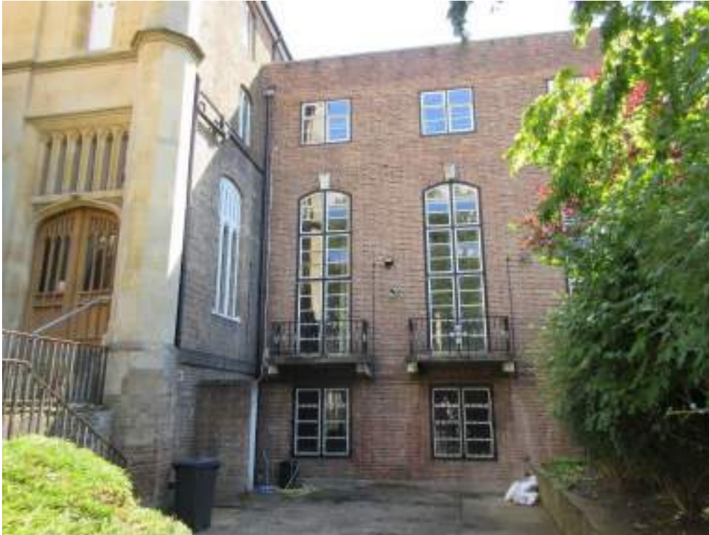
Figure 37: North-west elevation of north wing of the principal building and a glimpse of its rear (south-west) elevation, and the north-west elevation of rear extension A.
