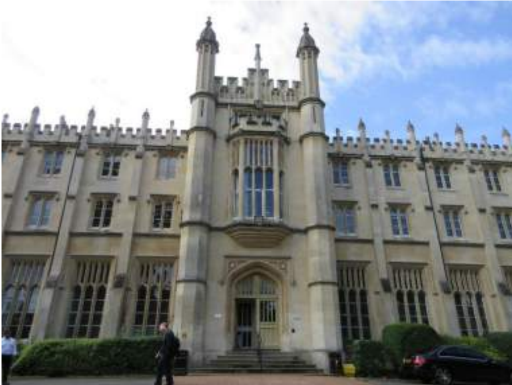
Figure 35: Front (north-east) elevation of the principal building.
