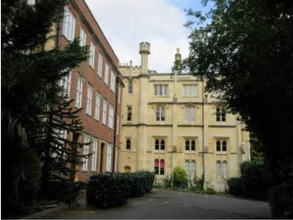
Figure 33: Side (south-east) elevation of south wing of the principal building, and a glimpse of the front (north-east) elevation of George House. The driveway/pathway is within the subject site.
