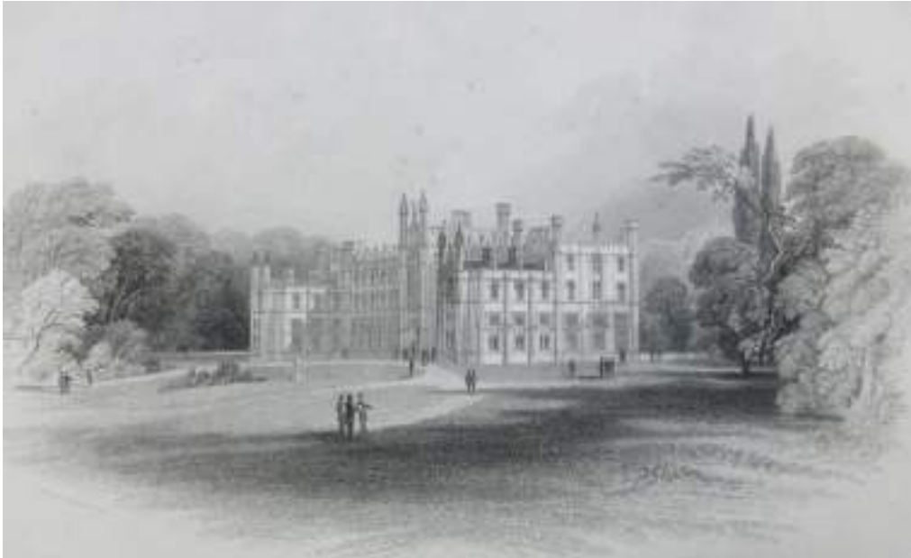
Figure 16: Undated print of the Wesleyan Theological Institution, showing the front (north-east) and side (north-west) elevations, and the surrounding landscape.
