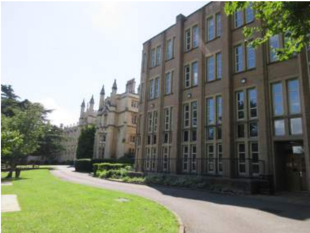
Figure 40: Southward view, with the principal building, and Sir Cyril Taylor Library (north-east elevation) on the right. The driveway/pathway is within the subject site.
