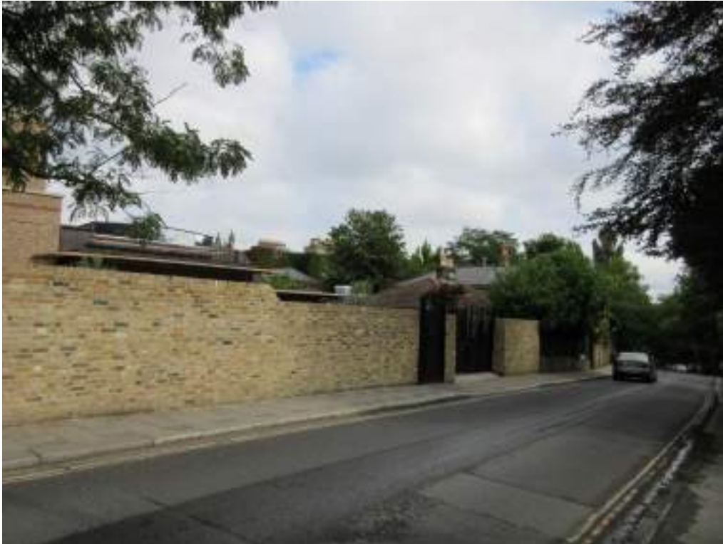
Figure 6: Northward view along Queen's Road, with glimpses of no. 3 (locally listed), and Upper and Lower Cottages (locally listed and curtilage listed).
