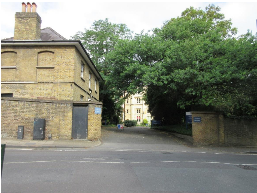
Figure 6: Westward view towards southern entrance to Thomas's College within RHCA. Lower Cottage (locally listed and curtilage listed) is on the left, and the principal college building (Grade II) is in the distance. Driveway is within subject site.
