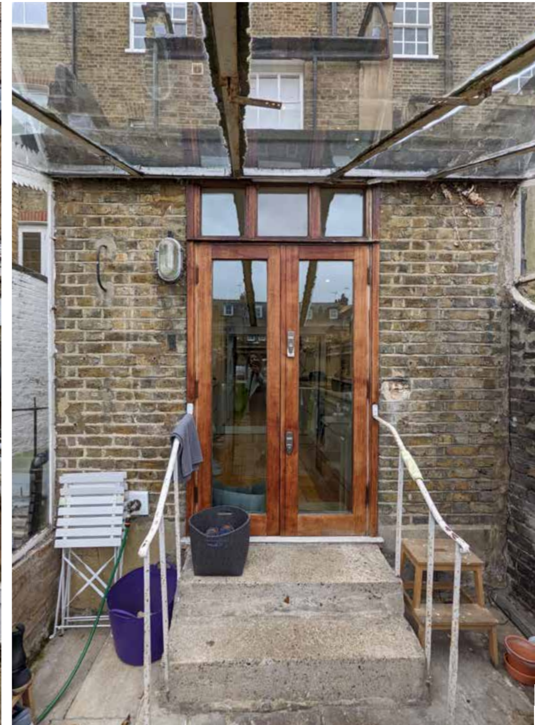
Internal view within conservatory of existing 'solid' closet wing structure behind
