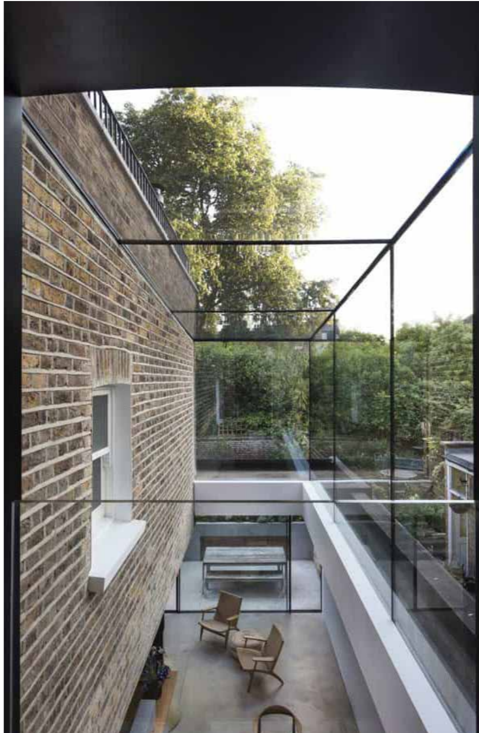
A double height glass infill extension to a Victorian property in the Kentish Town Conservation Area by Finkernagle Ross Architects successfully incorporates a lightweight, frameless structural glass enclosure to preserve the visual distinction between solid and void spaces
