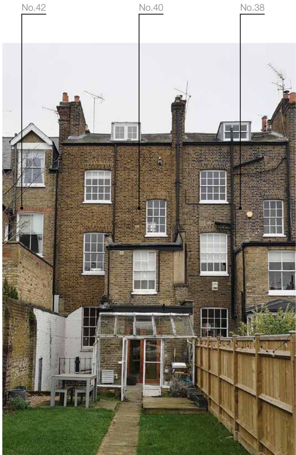
no.40 rear elevation with poor quality glass extension beyond enlarged closet wing view across rear of terrace cluster with varying sized closet wings, alterations and extensions
