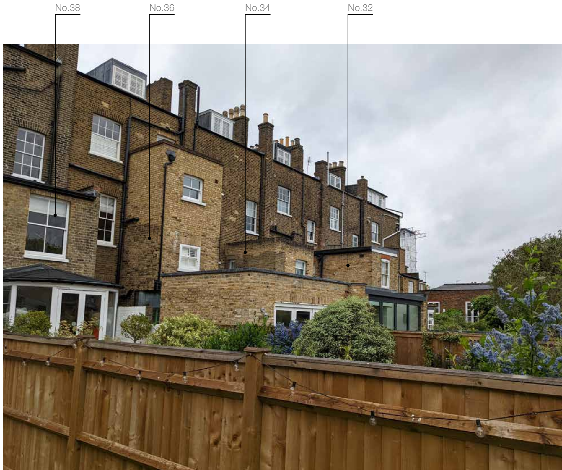
no.40 rear elevation with poor quality glass extension beyond enlarged closet wing view across rear of terrace cluster with varying sized closet wings, alterations and extensions
